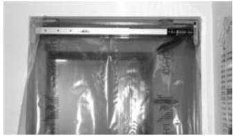
Figure 3: Properly installed Phoenix Quick chamber
